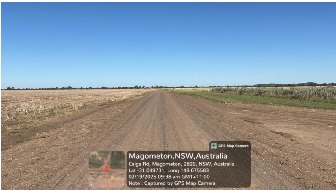
Figure 5: Natural disaster restoration work completed on Calga Road
