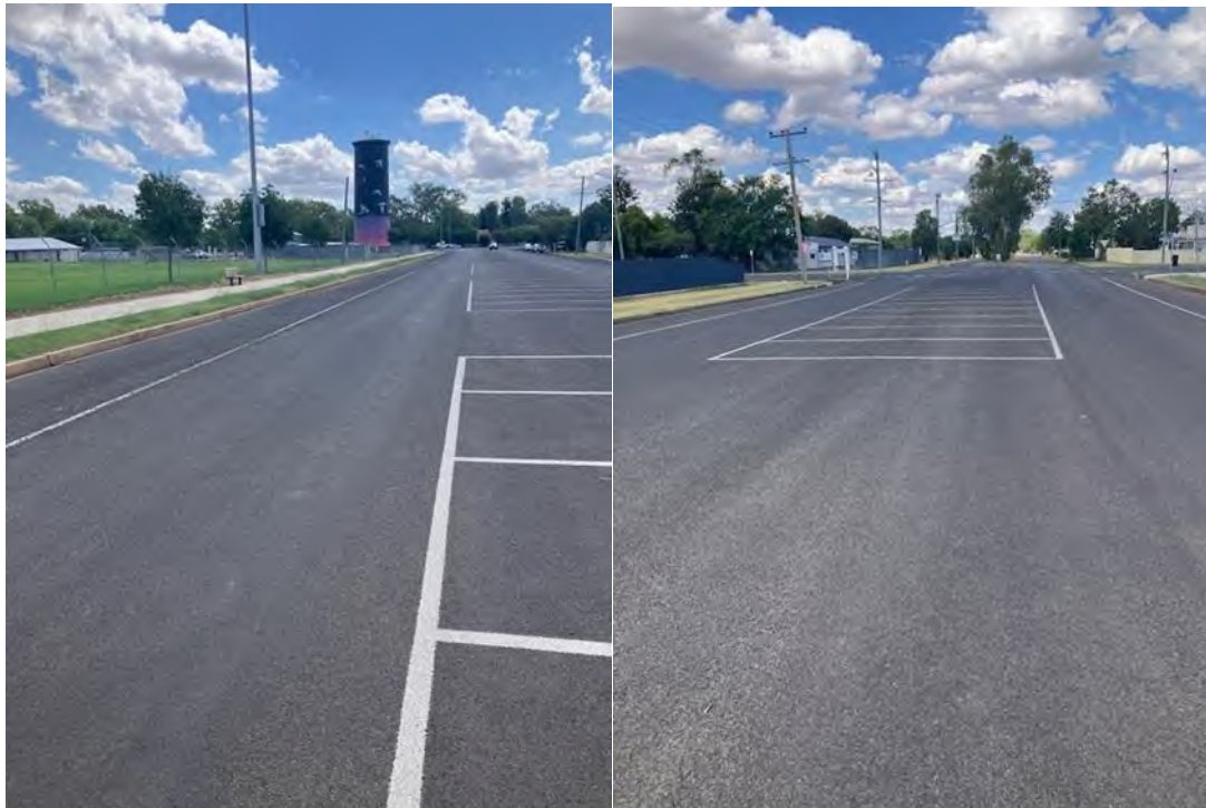
Figures 3 and 4: McCullough Street showing linemarking and location of centre tree planting
