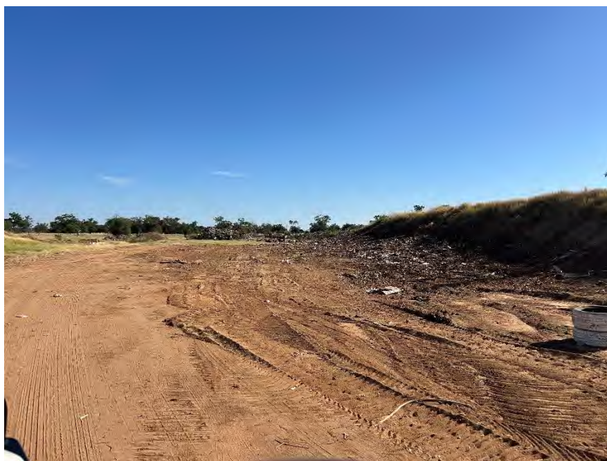
Coonamble after scrap metal removed on 28 Feb
