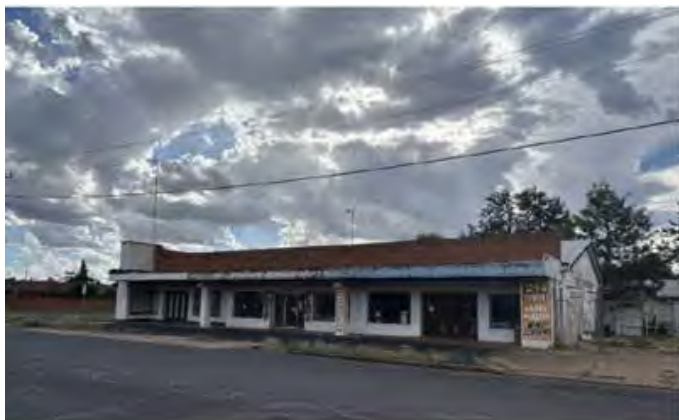
LEFT: Empty Town Shops in Nyngan
