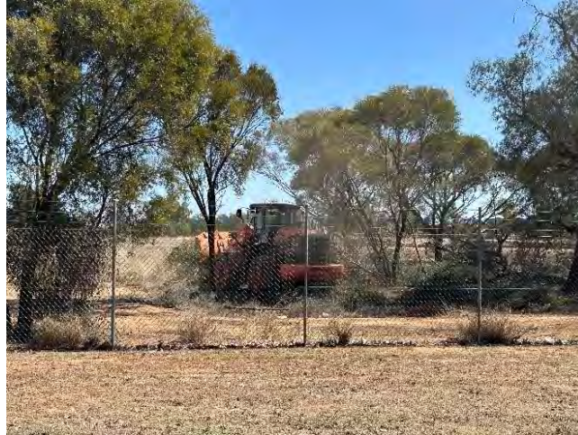
Plant operator training clearing the boundary fence line of windblown litter.
