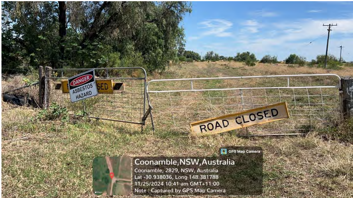
Secure site with fencing and signage.
