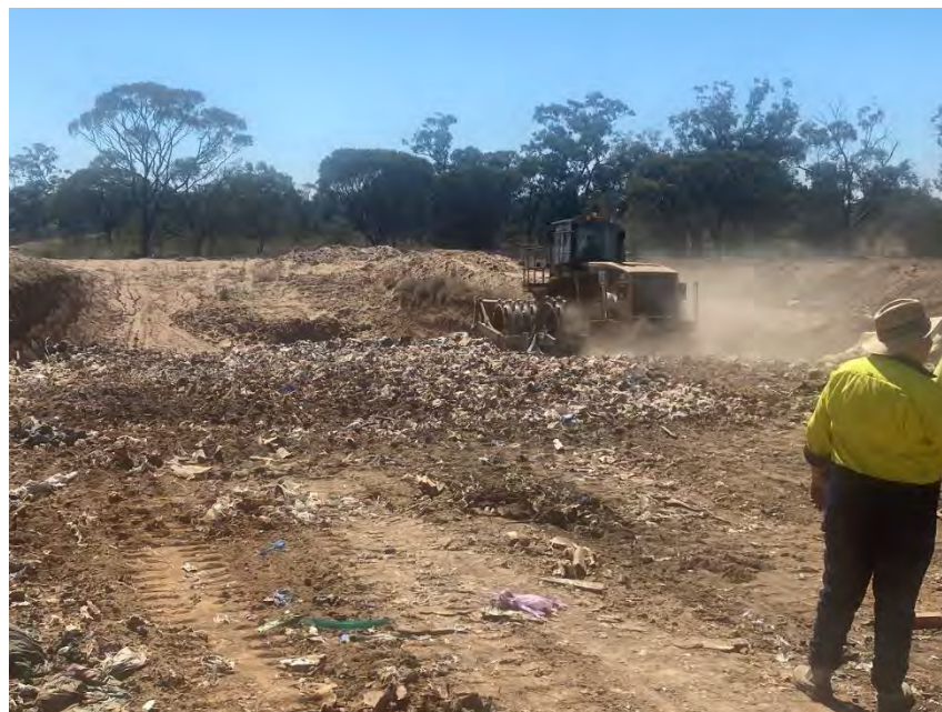
Compactor working on landfill
